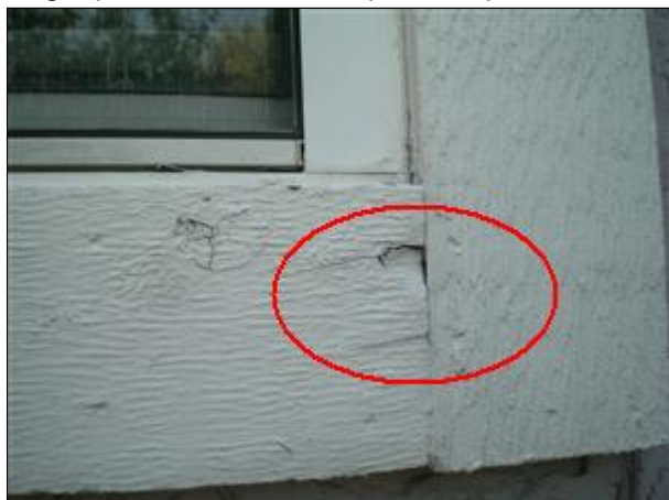
2.0 Picture 1 window at west side of house
